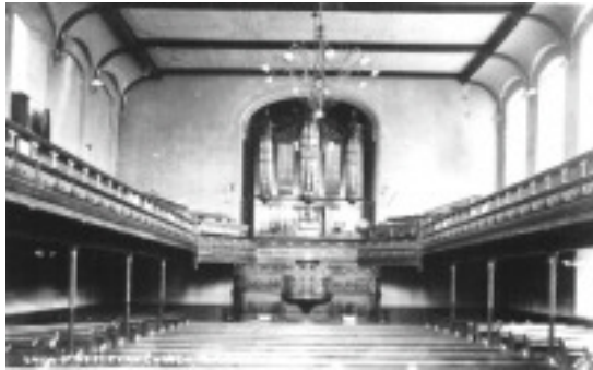
An interior view of the rebuilt Church
